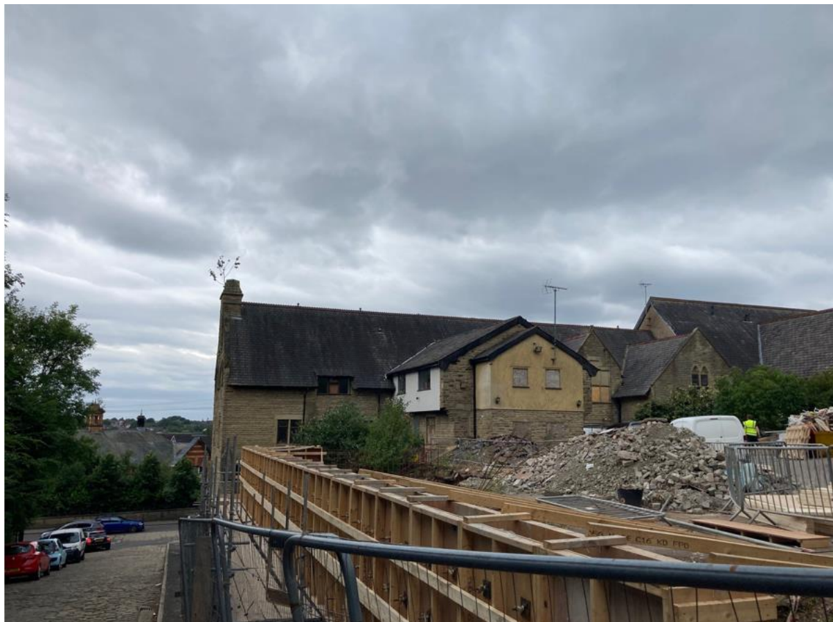
Photo 3: View of the rear portion of the site from Blandford Street (south eastern boundary)
